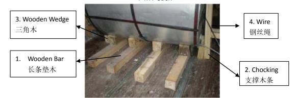
Put four wooden bars for each steel coil, and four stoppers for each Aft/Fore side. 每一卷下面垫放四根垫木,前后各需 4 个三角木固定
